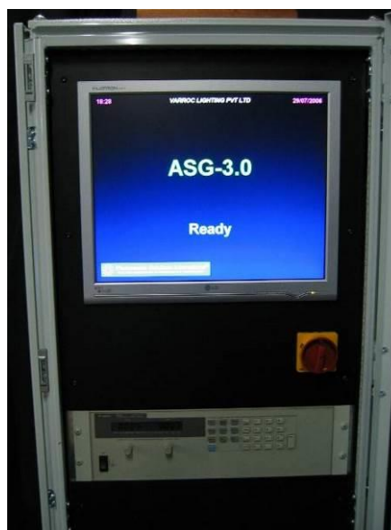
Figure 19: Secondary Display Mounted in Rack
