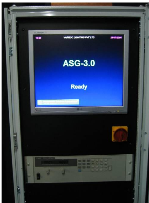
Figure 3: Professional Rack System
