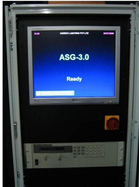
Figure 13: Secondary Display Mounted in Rack
